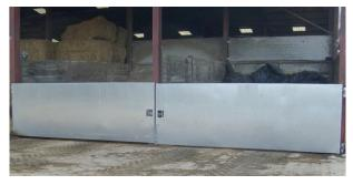
Fig.1: Sheeted gates across feed storage bays
