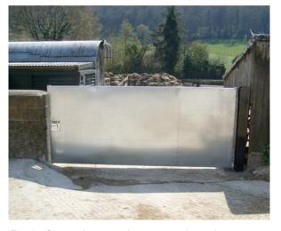
Fig. 3: Sheeted gate replacement to barred gate
